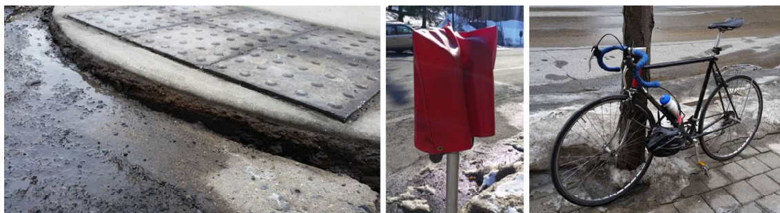
Fig. 17 Changes to the environment not modeled by the system. Winter conditions raised the curb cut out by 8 cm ( left ). A parking meter covered by a bag ( center ). A bike chained to a tree ( right )
